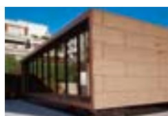
BTV Bank, Innsbruck, A Hanno Vogl-Fernheim, Innsbruck Spenglerei & Glaserei Anker, Hall TECU® Net Bronze
