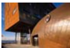
UEC – Urban Entertainment Centre, Almere, NL Will Alsop Architects, London Ridder Dak- en Wandsystemen BV, Hoorn TECU® Brass
